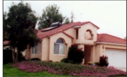
SunSiphon Installed on Tiled Residential Roof
